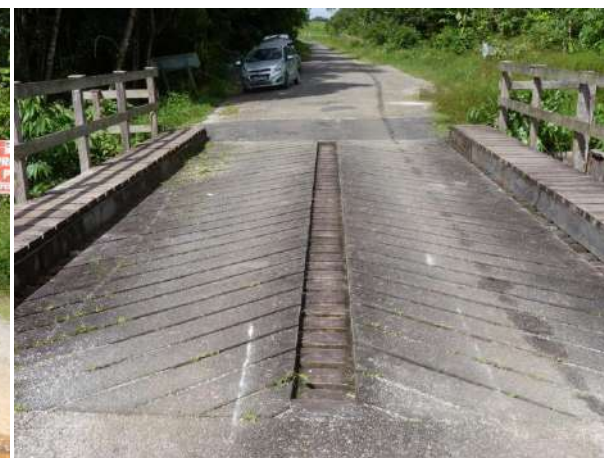
Figure 30: Pont, structure bois
