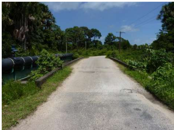
Figure 61: Pont, structure béton
