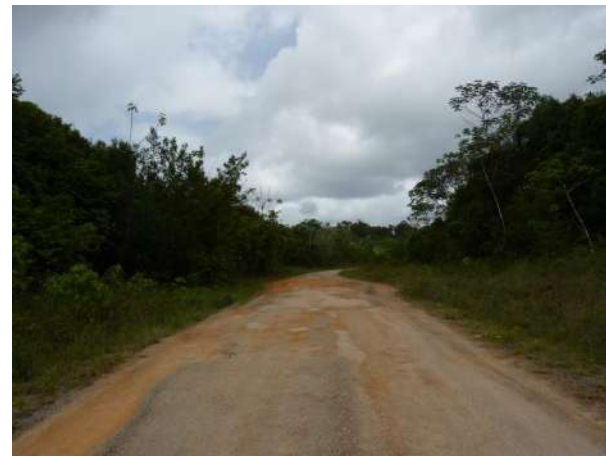
Figure 53: Elargissement de la route
